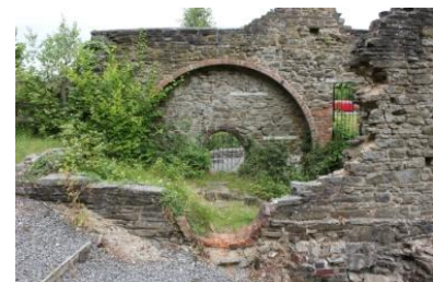
Snailbeach Crusher Building
