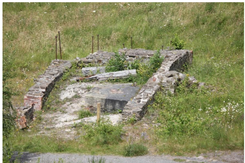
Foundations of the Halvans Building
