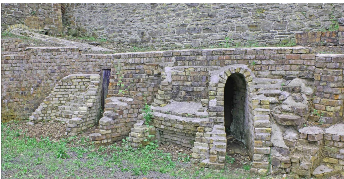
Remains of the Boiler House for the Compressor
